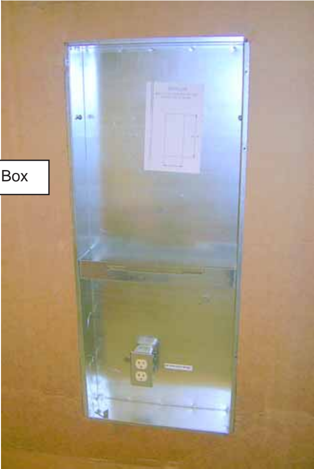
Installing ESWA unit onto ESRC Wall Box leaves exposed opening
